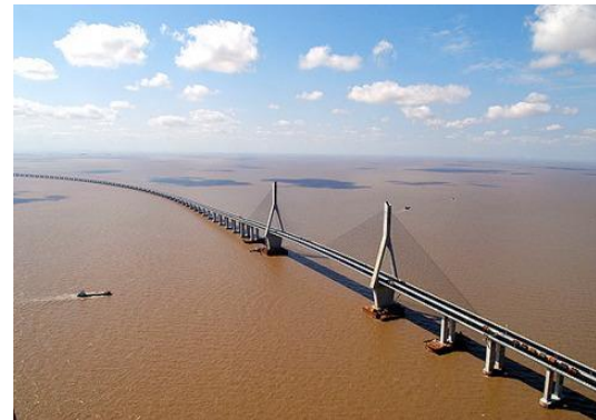
Fig 4: Donghai Bridge, Shanghai
