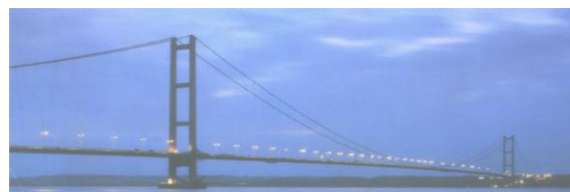
Fig 1: The Humber Suspension Bridge
